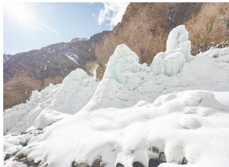
An artificial glacier built by Pakistani villagers during winter to provide water for the summer at Pari village in Kharmang district, Gilgit-Baltistan. – AFP/IC
