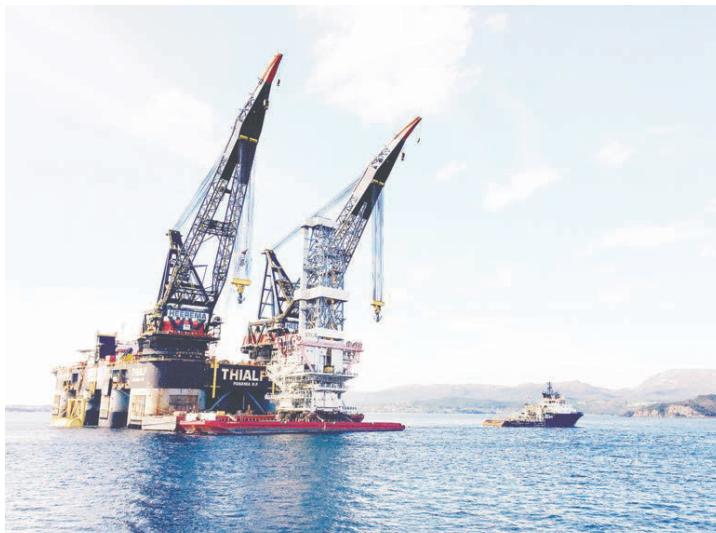
An oil drilling platform at the giant offshore Johan Sverdrup field near the municipality of Stord in western Norway. — REUTERSPIC
