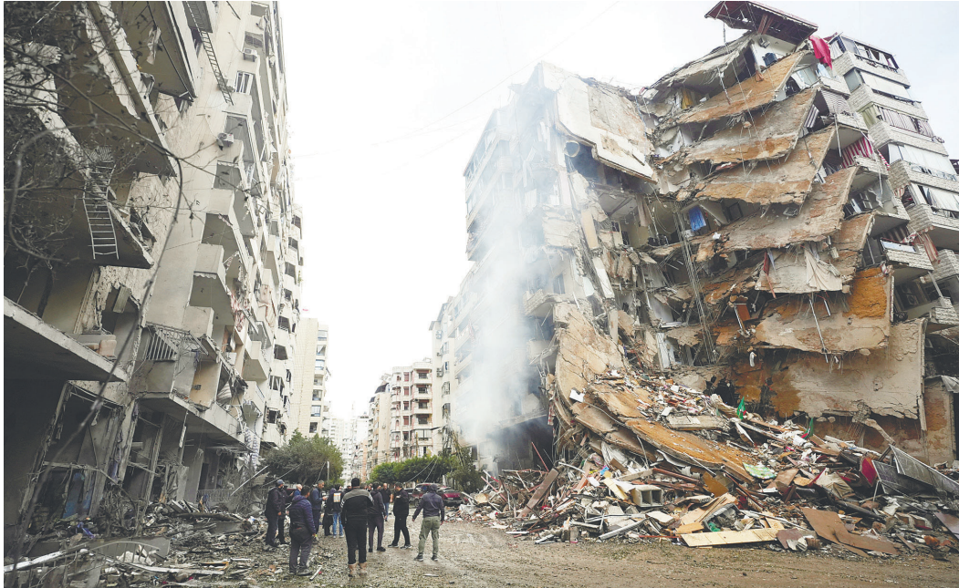
SENSELESS DESTRUCTION ... Residents walking past damaged buildings in the aftermath of Israeli strikes on Beirut's southern suburbs yesterday, amid ongoing hostilities between Hezbollah and Israeli forces. – REUTERSPIC
