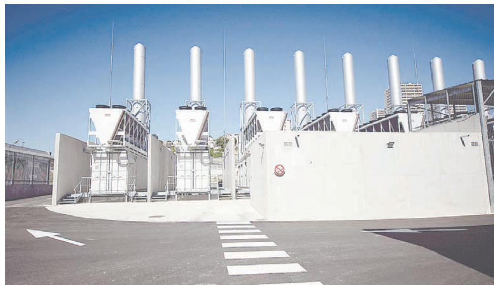
The portside data centres pump water at a rate of about 3,000 cubic metres per hour to keep servers cool. – AFP/IC
